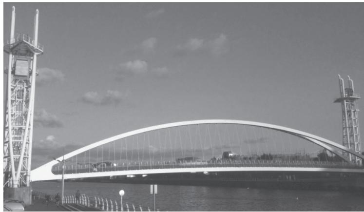
When large numbers of people cross the bridge at the same time, the bridge begins to oscillate with large amplitude simple harmonic motion.
